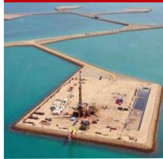
Aramco Manifa Gas processing plant
