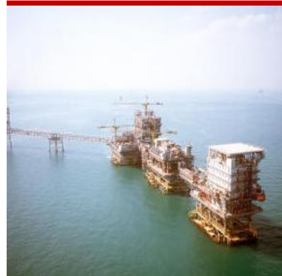
Aramco Karan Offshore Gas Platform
