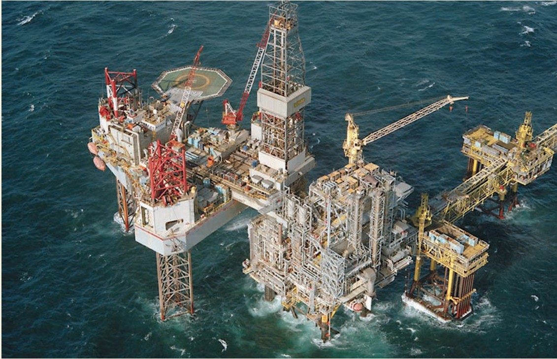
Ensko 71 of the Hitachi K1032N design. It was constructed in 1982 and modified in 1995. The rig location is in the North Sea, Denmark at a current water depth of 142 ft.
